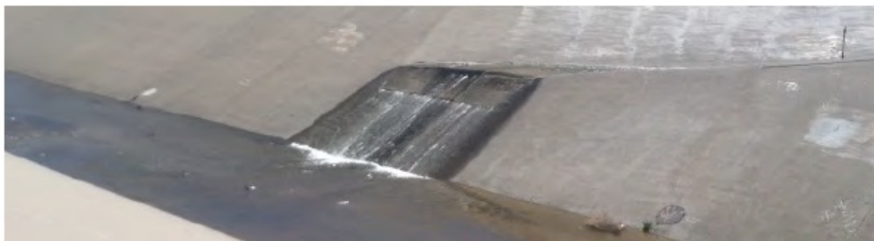
North Diversion Channel, Albuquerque, NM (photo by Tess Houle)
