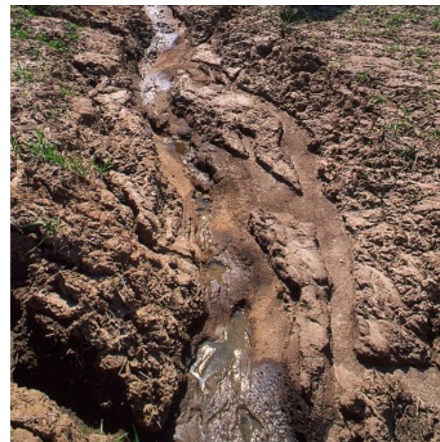
Signs of soil erosion
