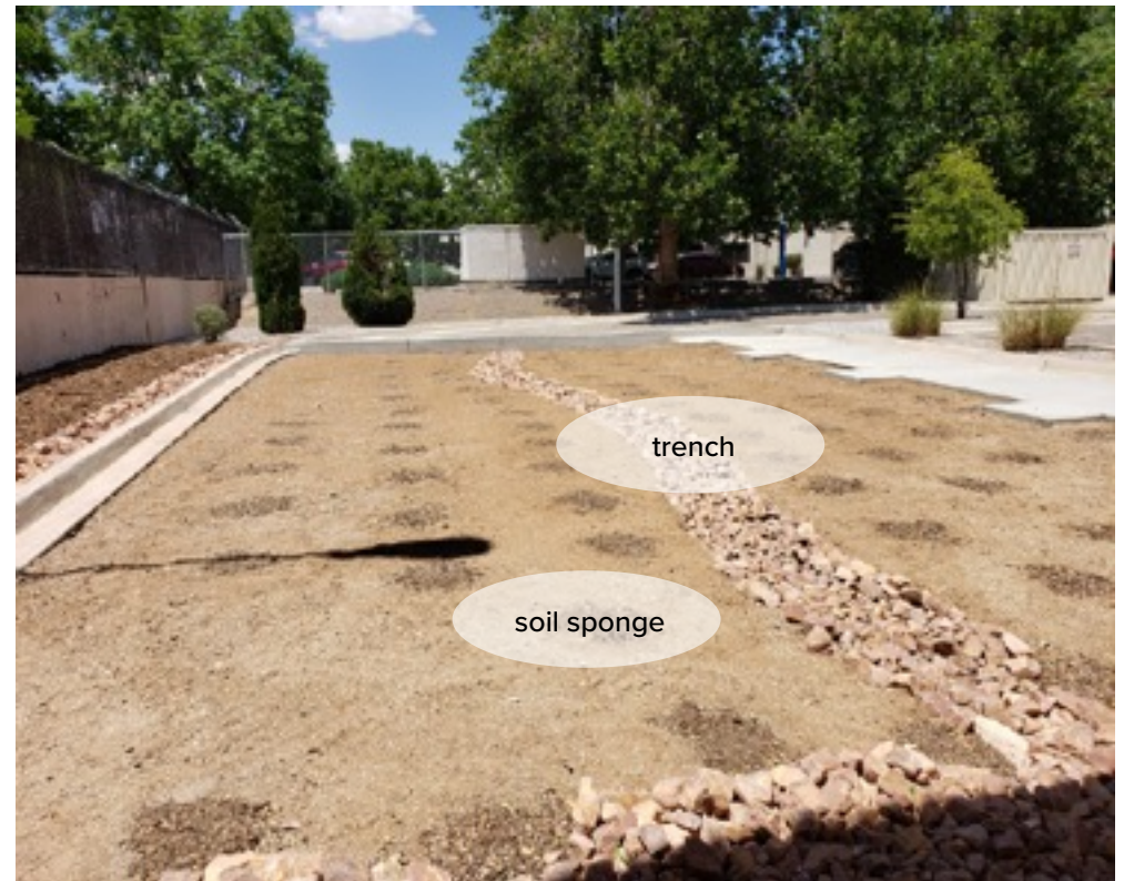
Urban agriculture infiltration conveyance including a conveyance trench and soil sponges.
