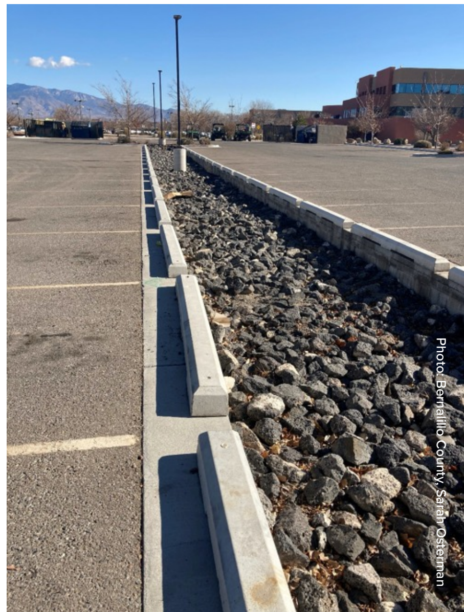
Infiltration trench in parking lot
