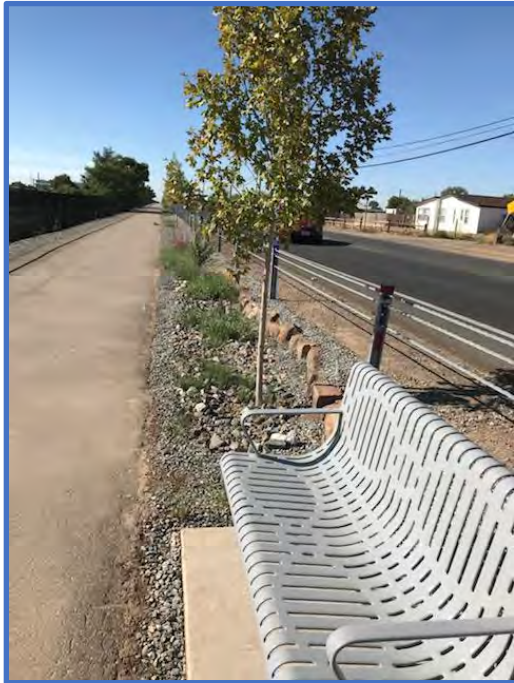
Figure 2: Example of Rural Type Road with Bioswale
